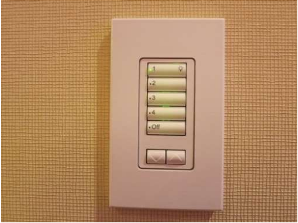
The Keypad offers a user-friendly front-end interface to activate preset scenes.
